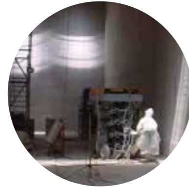
Vandellós I NPP dismantling: Decontamination of concrete walls.
